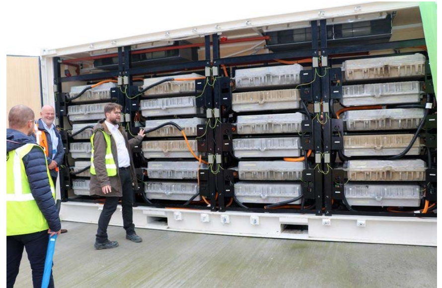
Second-life battery units (coming from Renault-Nissan) – pilot at Umicore
